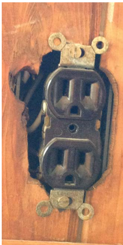
Openings around outlets often let cold air in, but drafts can be prevented by inserting a pre-formed outlet insulating cover which goes unseen once outlet plate cover is put in place.
