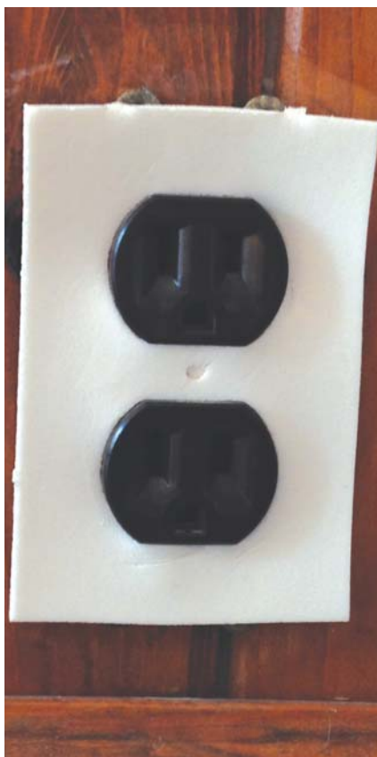
Openings around outlets often let cold air in, but drafts can be prevented by inserting a pre-formed outlet insulating cover which goes unseen once outlet plate cover is put in place.
